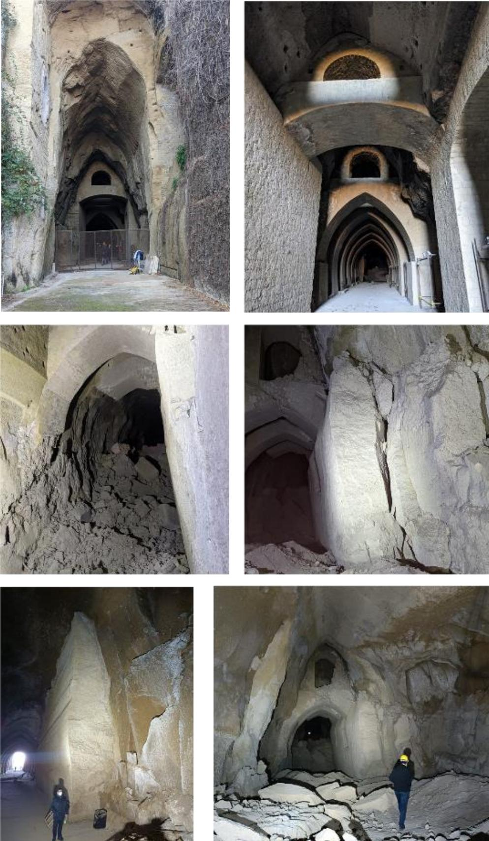
Figure 30. From top left: pictures from the eastern entrance till ca. progressive 150 m. Masonry arches well preserved in the first part, with complete collapse of side walls in the final part. Large subvertical rectangular blocks sometimes on the verge of instability failure.
