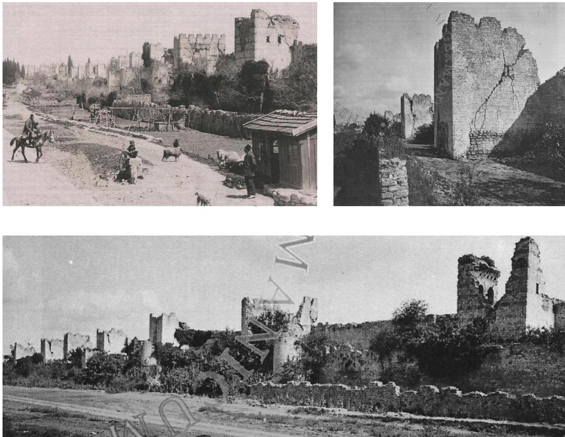
Figure 37. State of decadence of the Theodosian walls in the early 20th century, with clear evidence of unrepaired seismic damages to the towers (German Archaeological Institution, 1939).
