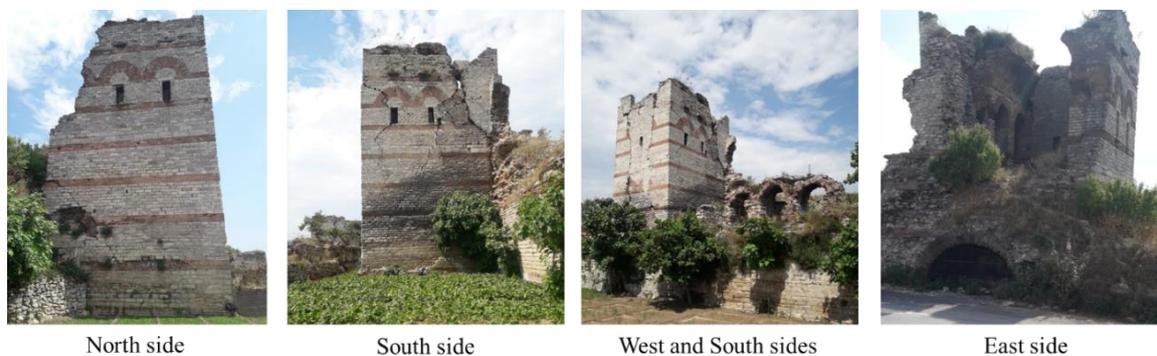
Figure 40. Recent views of all sides of tower 19. The damages caused by 1999 Kocaeli earthquake are clearly visible.
