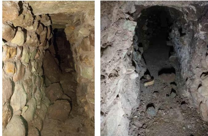
Figure 17. Examples of local collapses: (left) at the interface between lined and unlined stretches; (right) in an unlined tunnel excavated in fine yellow sand (*girín*) (modified after Lacombe *et al.*, 2020).
