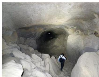
Figure 29. From top left: pictures from the western entrance till ca. progressive 350 m. Collapse of blocks, tension cracks and collapse of masonry lining are clearly visible;
