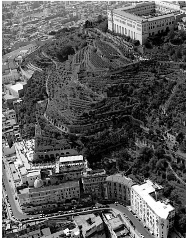
Fig 7. Bird's eye view of the Vineyard, with part of its retaining structures
